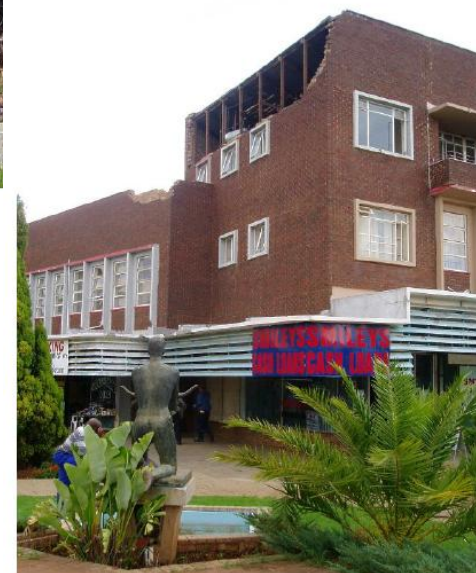
Example of damages caused by the post-mining EQ in Stilfontein in 2005, Durrheim et al. 2007
