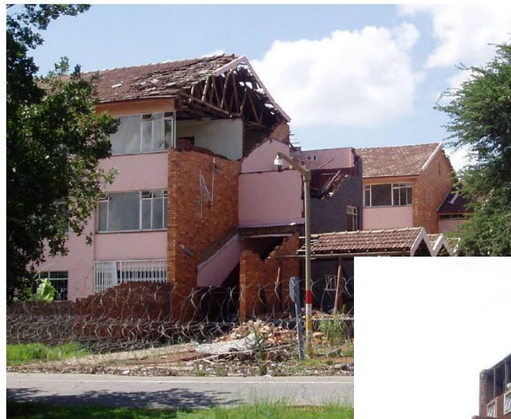
Example of damages caused by the post-mining EQ in Stilfontein in 2005, Durrheim et al. 2007
